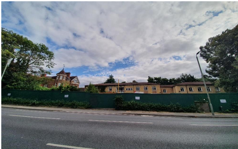
Image 3: Frontage of application site.
